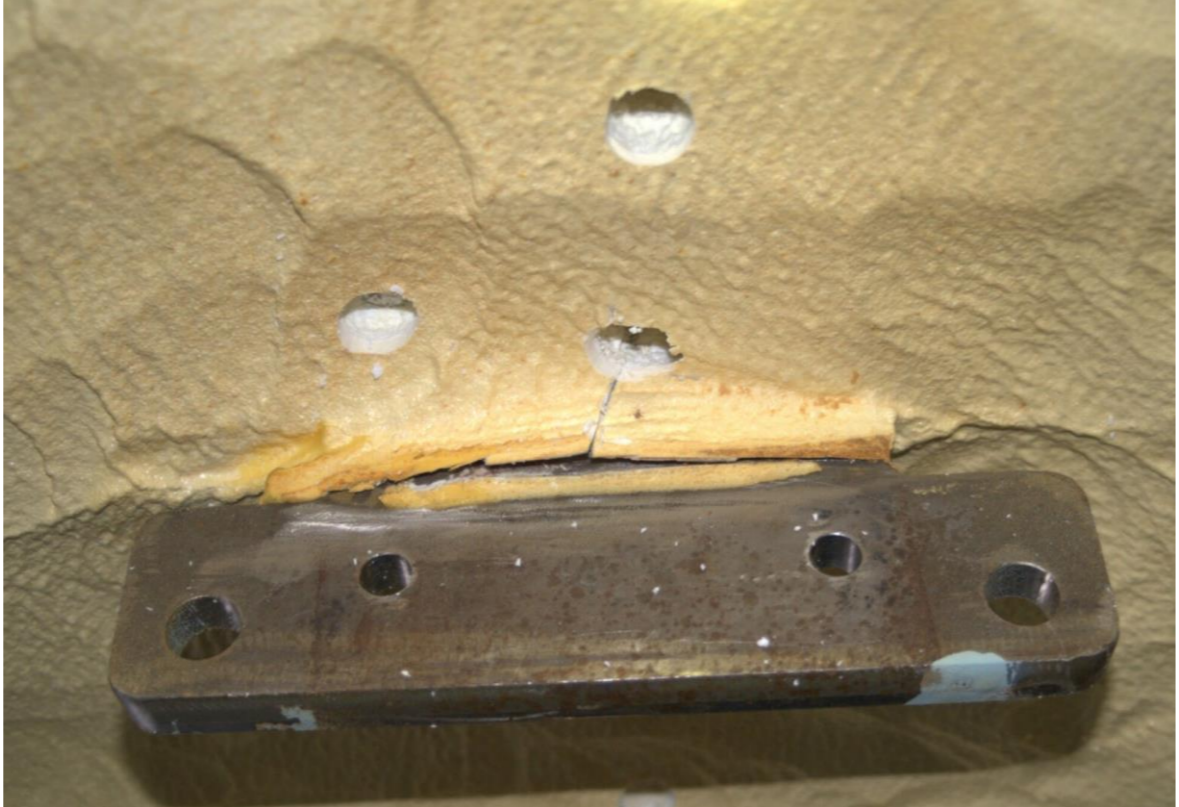
Anchor point good. No degradation of structure
