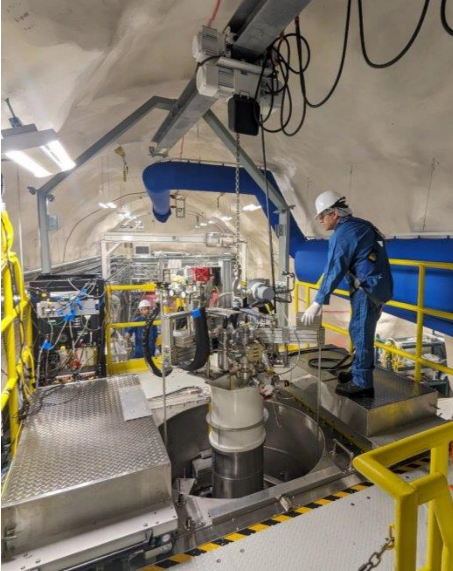
Lowering of DR into drywell
